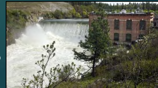
Nine Mile Dam, Avista Corp
